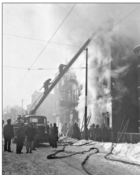
Two alarm fire at the Quality Bakery, 2952 S. Wallace, 12/27/1950
