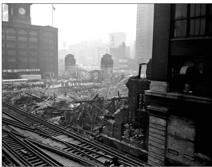
Ruins of a waterfront warehouse at 320 North La Salle, 1/12/1951. Firefighters Jack Schuberth, Henry Dyer, John Gleason, and Patrick Milott died when exploding drums of lacquer thinner collapsed a wall of the four story building on them. 25% of the CFD responded to the fire.
